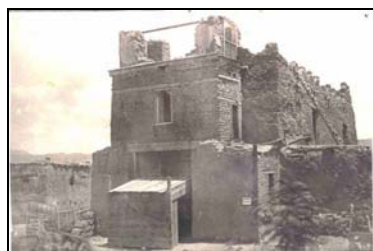
San Miguel after bell tower collapse in 1872.
