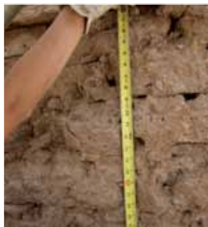
Making adobe bricks, the scaffolding, revealing the adobe behind the stucco
