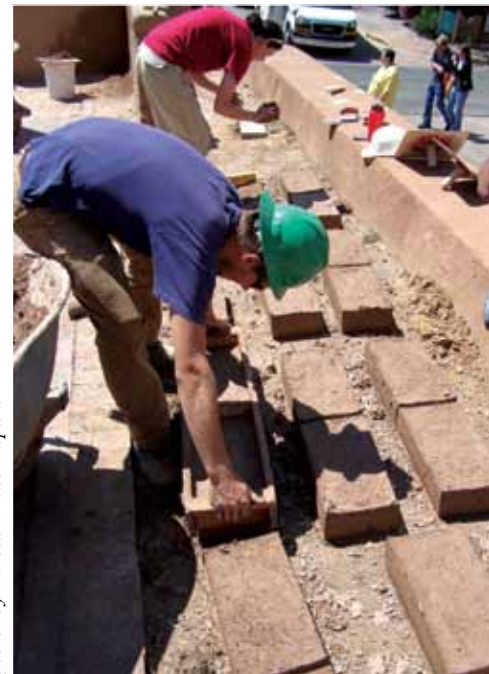
Making adobe bricks, the scaffolding, revealing the adobe behind the stucco
