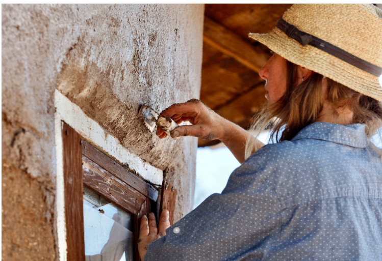
Don Sena, Project Manager, repairing capping on the parapet of San Miguel Church, Santa Fe, NM (right)
