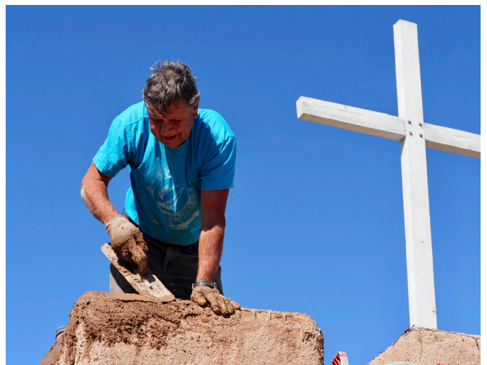
Don Sena, Project Manager, repairing capping on the parapet of San Miguel Church, Santa Fe, NM (right)
